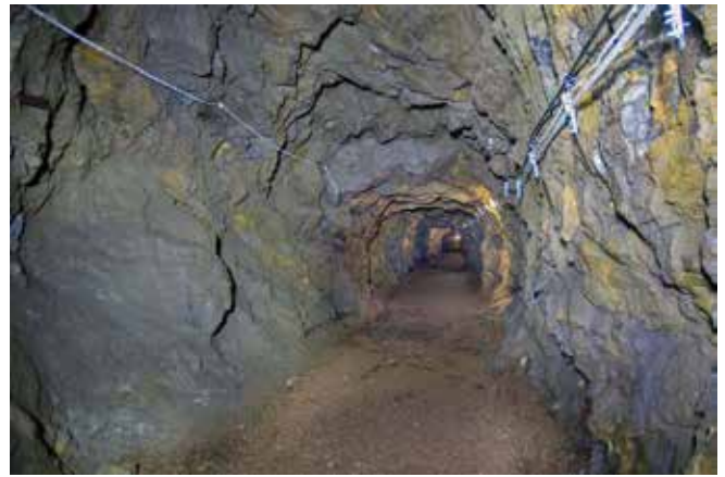
Crudely cut pilot tunnel at Wlodarz. Photo Chris Rayner
